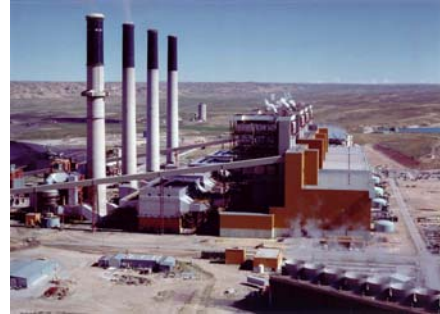
Jim Bridger Power Plant – Point of Rocks, WY
